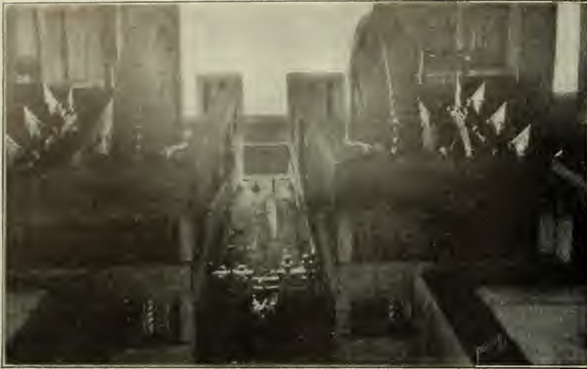
FIG. 3. CONVEYERS AT THE TOP OF THE WASHERY
